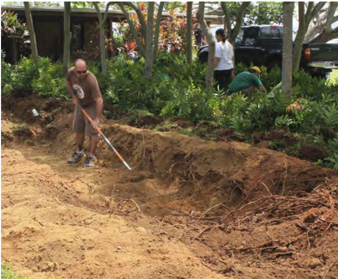
Left: Excavate the rain garden to the proper depth with hand tools and volunteers.
